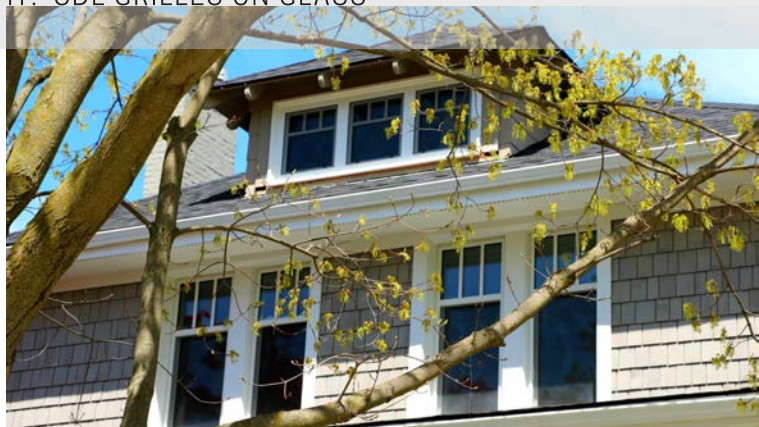
TOP: TRIPLE GLAZING WITH LOE366 LEFT: DUAL GLAZING WITH ACID ETCHED PRIVACY GLASS RIGHT: SDL GRILLES ON GLASS
